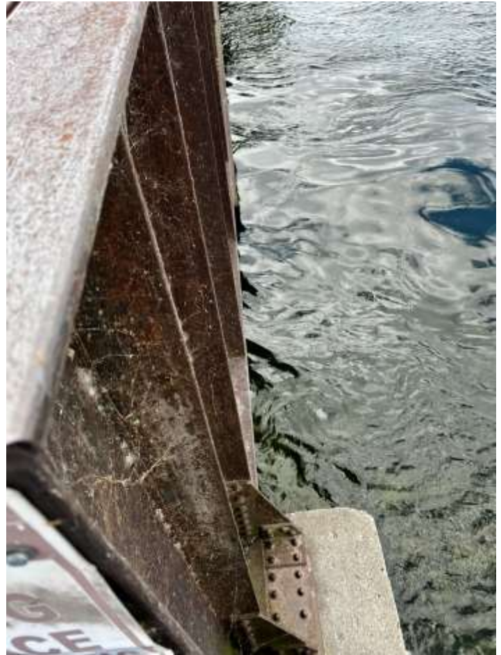
I-beam visible by leaning over the Colchester Causeway bridge railing. • Photo courtesy Kari Jo Spear.
